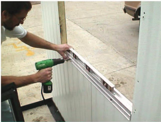
Figure 3 (viewed from interior)
